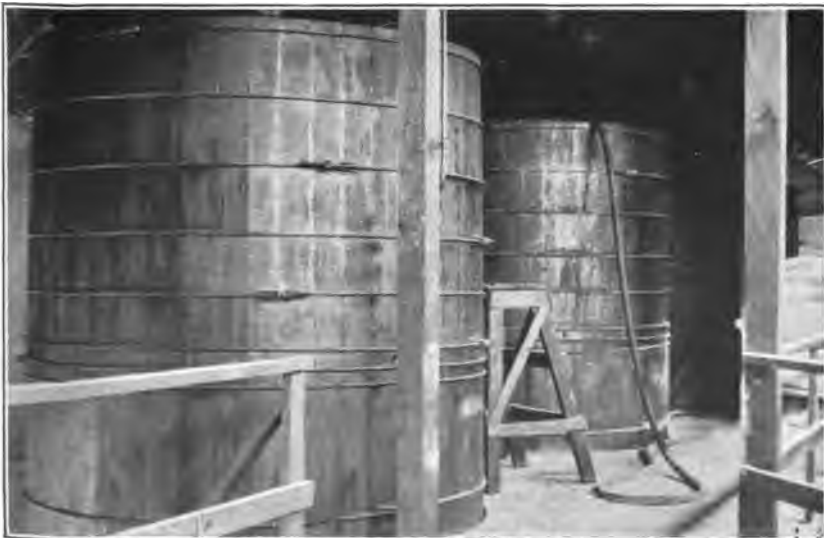
B. UPPER PART OF SETTLING TANKS, SHOWING FLOATING SIPHON.
